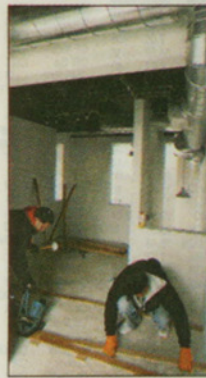
Workers Fernando Hernandez, left, and Jovanny Montalvo lay hardwood flooring.
